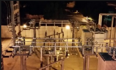
(a) Image Pipes.BB, MOS: 2.810
